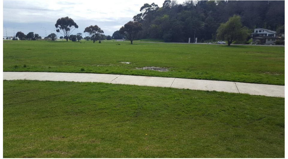
Evidence of Surface Water Pooling
