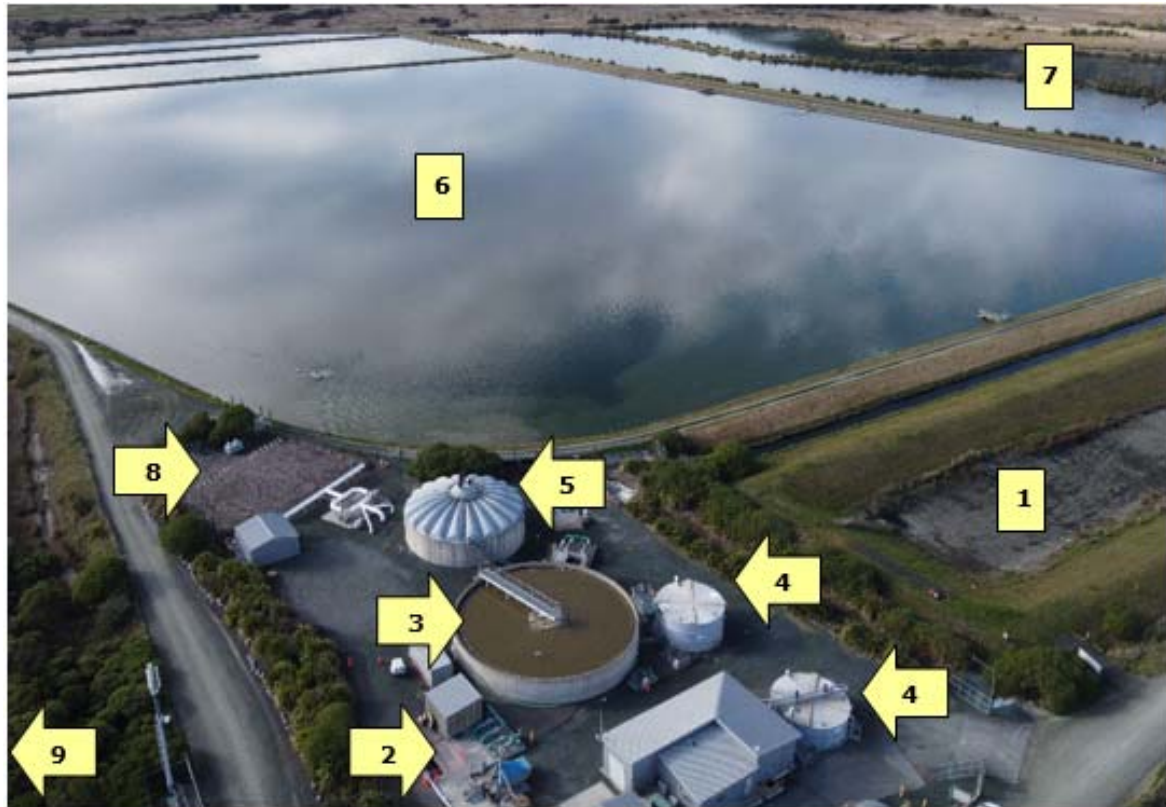
Figure 4-8: Nelson Wastewater Treatment Plant
