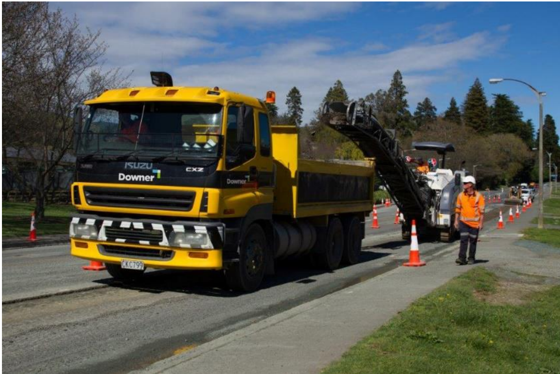
Figure 8.1: Pavement Resurfacing Project
