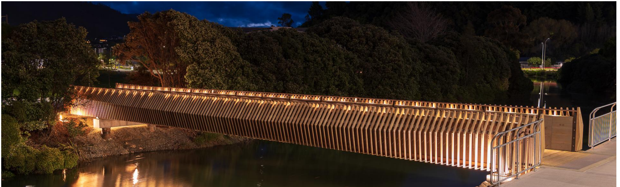
Figure 63 - Salt Water Creek Bridge
