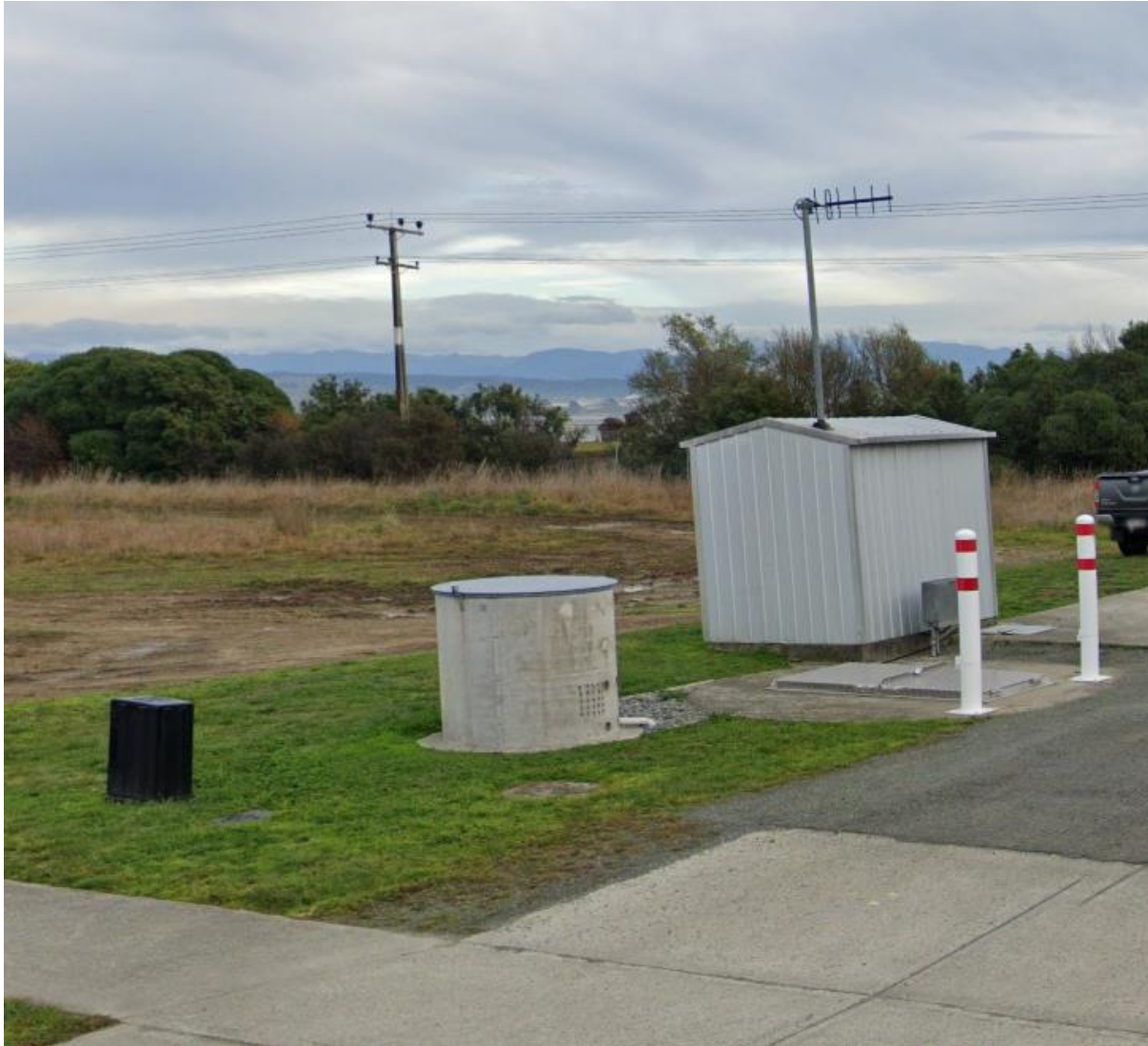
Figure 7-3: Photograph of the Whakatū Pump Station site
