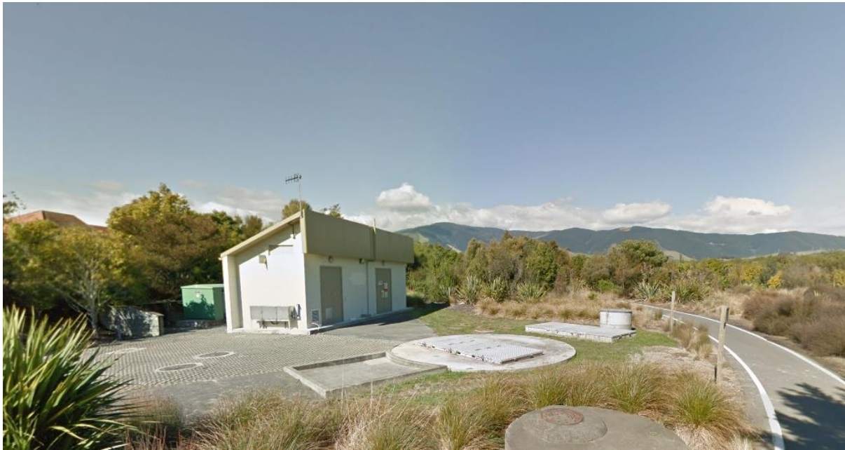
Figure 7-7 Photograph of Songer Street Pump Station site
