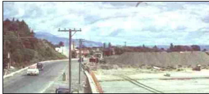
Fig 21: Stockpile during Rocks Road upgrade in 1958/9. (G. Toynbee)
