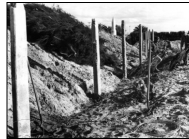
Fig 20: 1965 erection of brushwood fences to protect the carpark and playground. (Nelson Provincial Museum: Geoffrey C Wood collection L6176 fr 8)
