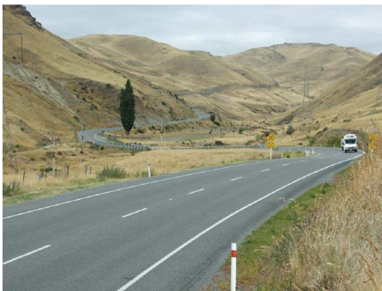
Puka Puka Weld Pass SH1, Marlborough
